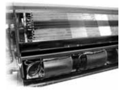
Figure 17: Fan board removal for fan/ motor access
